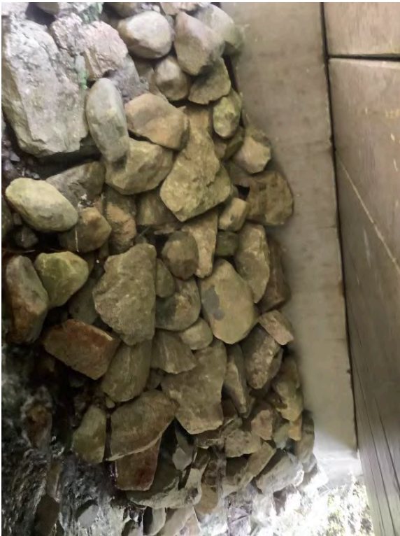
Left Bank Abutment when facing downstream
