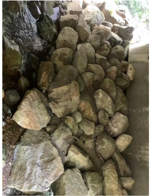
Right Bank Abutment when facing downstream
